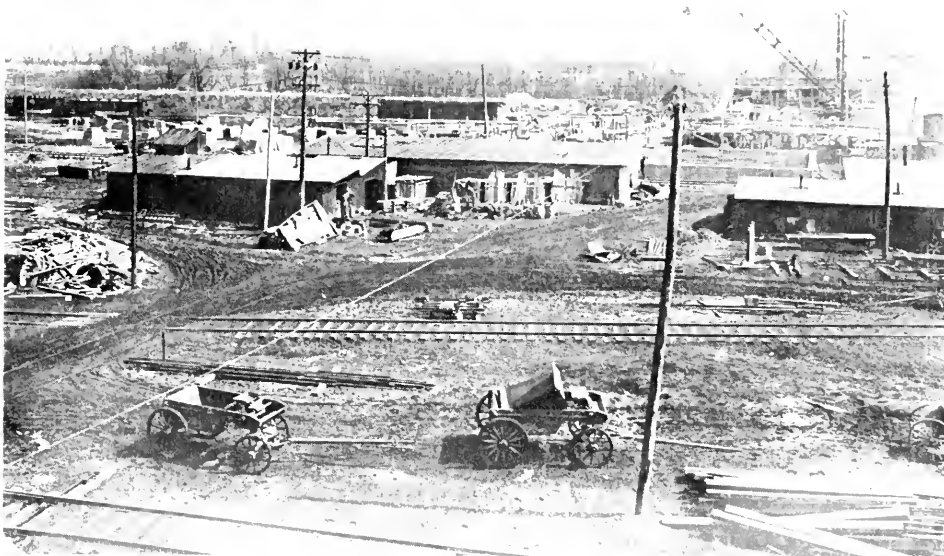
Keystone's Steel Mill under construction in 1917
